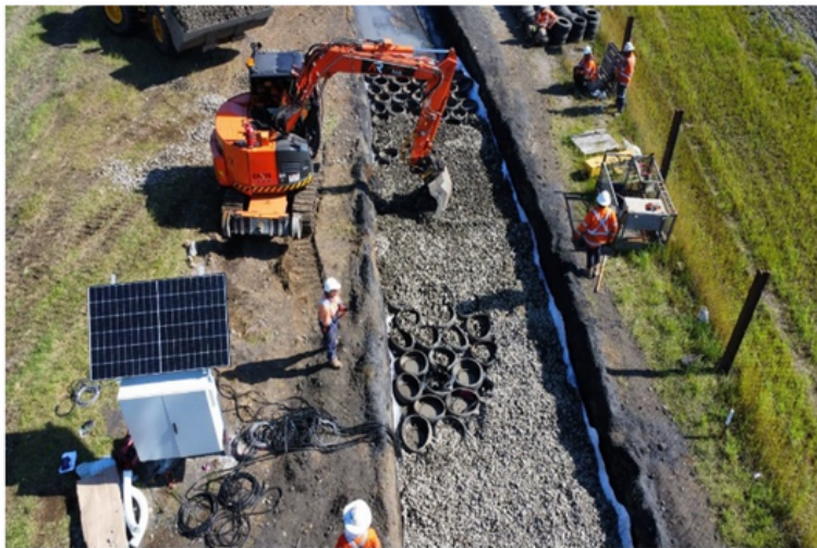
Figure 6: Construction of a railway track using recycled waste
